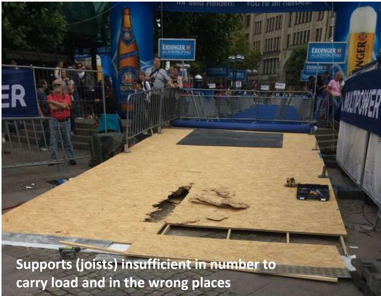
**Supports (joists) insufficient in number to carry load and in the wrong places**
